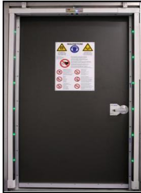
Figure 1: The ferromagnetic detector lines the door into the scanner room.
